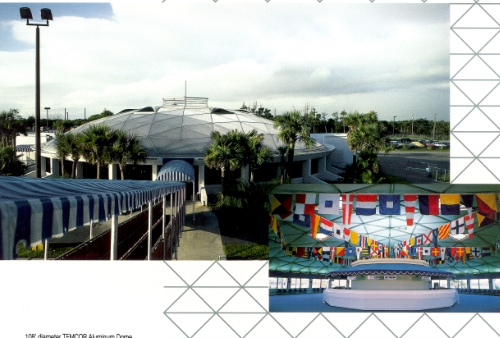
108' diameter TEMCOR Aluminum Dome
